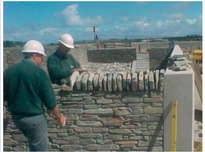
▲ The emergency workforce used local stone wherever possible
