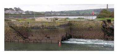
added at the time of the installation of the pipe line to the North Quay [1940] to help keep water back for water extraction (see CQ15). There are the remains of concrete control house on the top of the structure.
