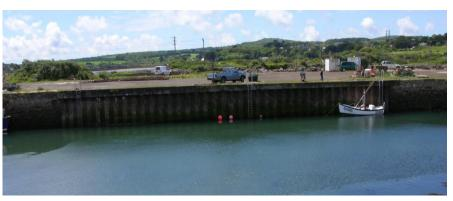
just beyond the collapse – it is because of the poor state of the wall partly due to the possible internal collapse of the tunnel (SQ16). There is a set of stone steps down to the water at the extreme north west corner.
